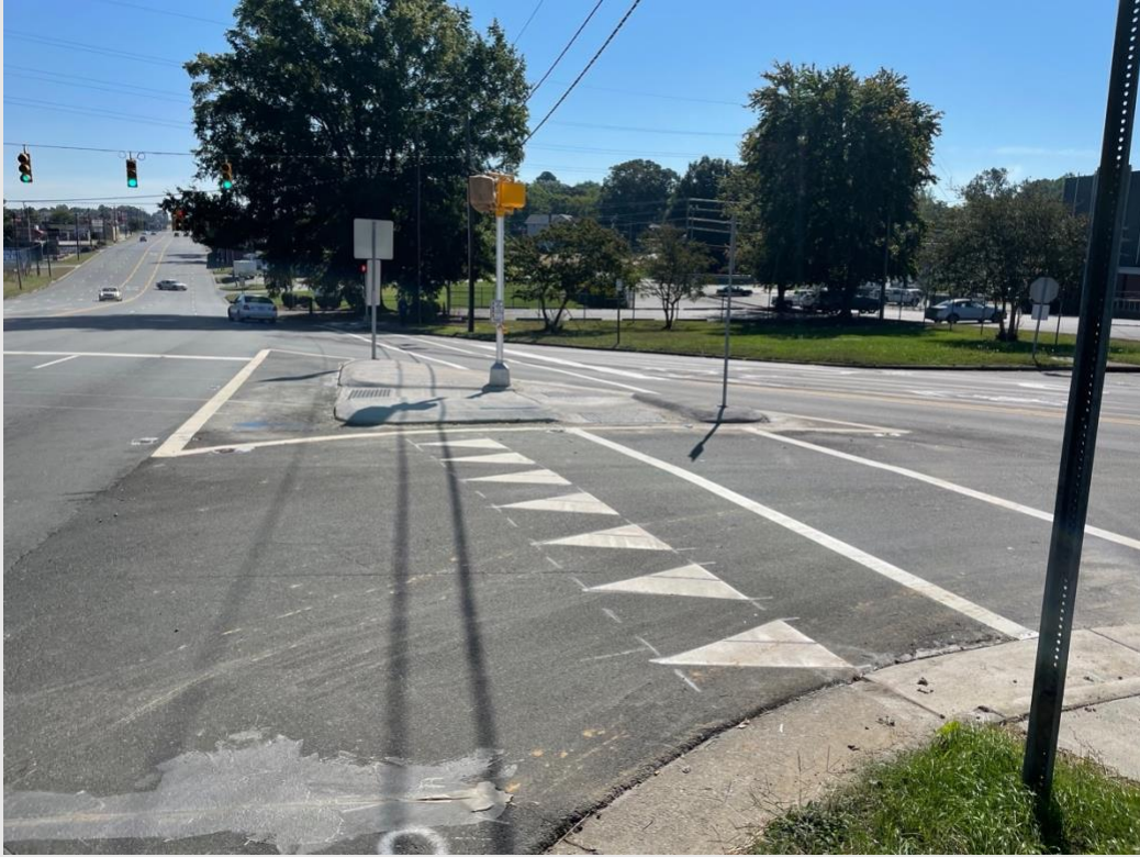
Image 13: Pedestrian crossing at Main Street and North Church Street looking east
