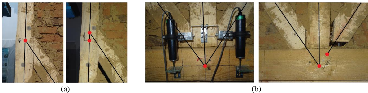
Figure 8: Vertical sliding along the post (a) and detachment along the diagonal axis (b): initial and final position
