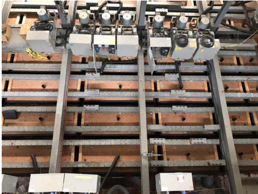
Figure 3.7: Installing pressure chambers.
