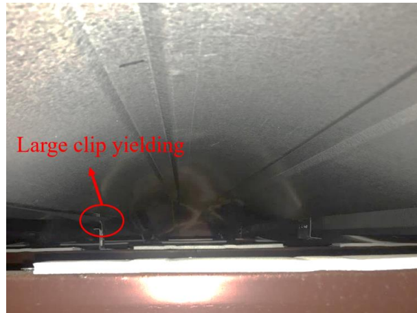
Figure 4.8: Deformation of panels under high uniform pressure.
