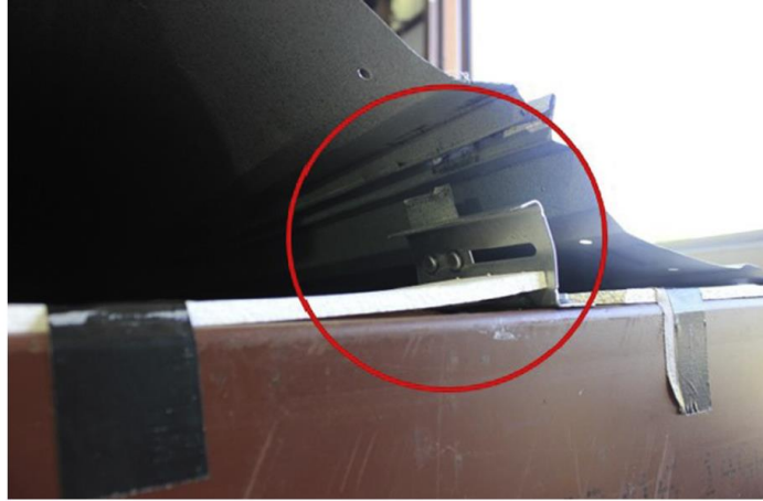
Figure 2.13: Seam to clip separation (Habte et al., 2015).
