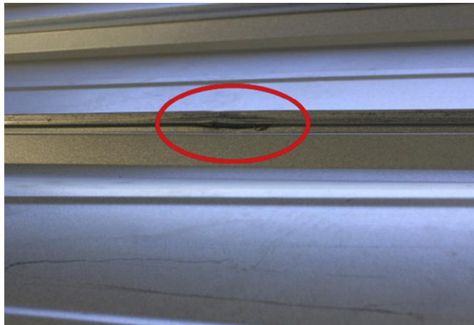
Figure 2.14: Initiation of seam disengagement (Habte et al., 2015).
