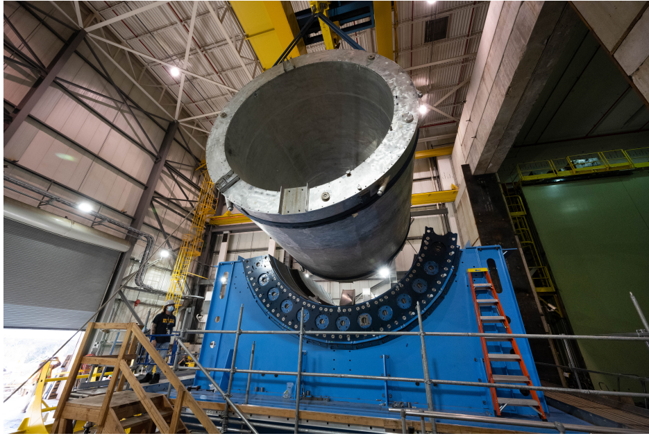
Figure 7.14: Installation of the BABAR magnet into the sPHENIX cradle.
