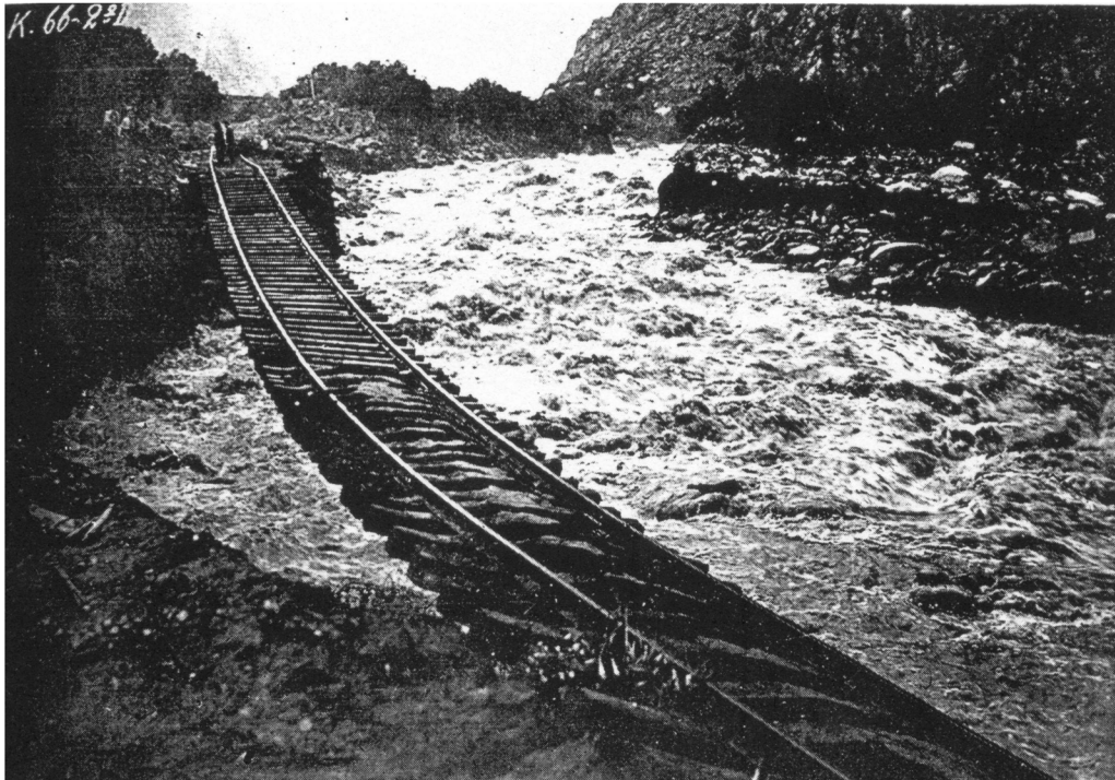
Illus. 22: Flood damage to the Central Andean Railway during the torrents of 1925 along the Río Rímac (illustration: BCAG 2:3 [1926]).
