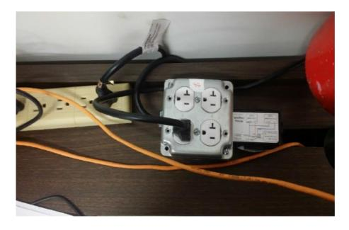
FIGURE 14: Enlighted Plug Load Controller installed at ECS 411.
