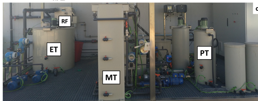
Figure 1. DM pilot-plant: (a) diagram scheme, (b) membrane module scheme and (c) picture.
