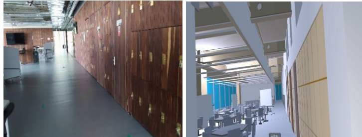
Figure 10 - Hallway 11th floor
