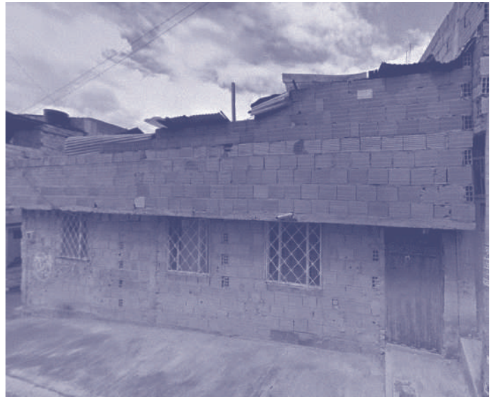
45. House under construction
