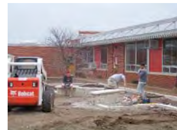
Figure 10. Contractors complete a stone bench begun by volunteers. Image by Kingery-Page.
