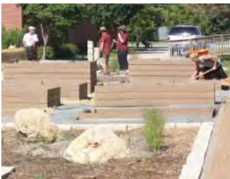
Figure 13. Volunteers spreading crushed limestone gravel. Image by Hunt.
