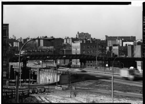
Figure 2. Cross Bronx Expressway: looking northwest at Third Avenue elevated over the expressway, 1973. Taken by Jack E. Boucher for the Historic American Engineering Record's archive (public domain).
