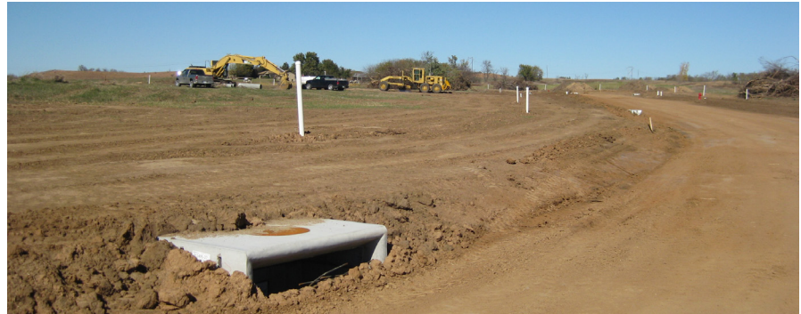
Figure 2.9 Road preparation and catch basin. Author 2010
