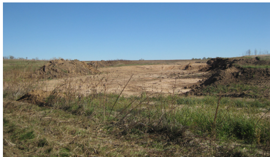
Figure 1.7 Borrow pits. Author, 2010
