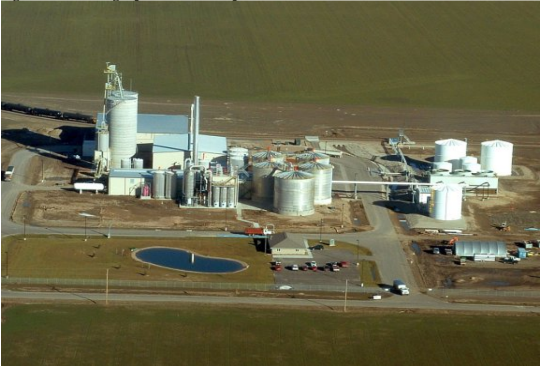
Figure 2.2: Photograph of site after plant was built
