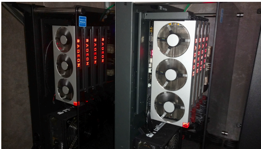
Fig. 3. Distributed system with two compute nodes incorporating four AMD Radeon VII each one.
