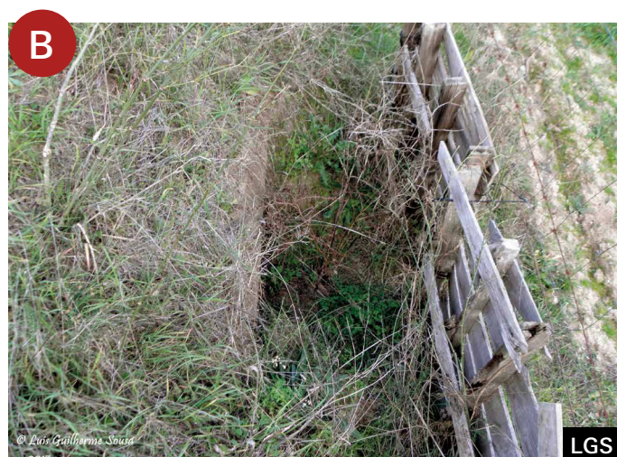
Examples of incorrect installation of fences: (A) gap between the fence and the passage wall; (B) fence placed in front of the culvert, with pallets hindering access to it.
