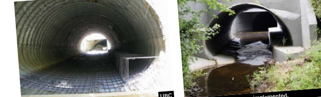
Building of the dry ledge and final aspect, in one of the culverts where this solution was implemented.
