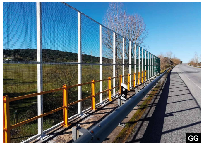
Details of the 3 m-high barriers implemented on the national road 114 road, made of rectangular-section metallic posts (RHS 80x60x3 cm) inserted in the foundation and topped by plastic caps, 2 m apart, that support a galvanised wire mesh welded and plasticized with PVC/polyester, with a 19 x 19 mm of diameter and a wire diameter of 2 mm.
