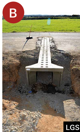
Works to implement permanent concrete barriers guiding animals towards the culvert.
