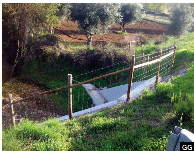
Examples of fences contouring the upper part of culverts, thus leaving their entries accessible.
