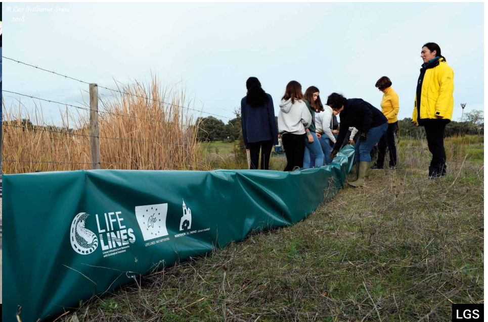
Installation of the temporary canvas barrier in the framework of the LIFE LINES project: (A) placement of the support structure, and (B) final aspect of the installed barrier.
