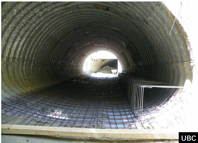
Building of the dry ledge and final aspect, in one of the culverts where this solution was implemented.
