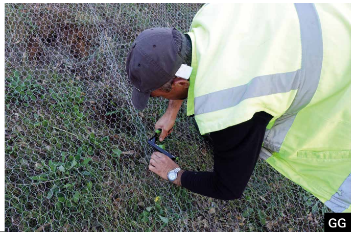
Installation of a deterrent mesh for rabbits on the road slopes of national road 4, Évora district.
