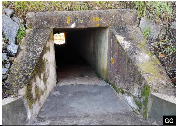
Adaptation of a rectangular culvert in the framework of the LIFE LINES project, by creating an entrance ramp and connecting it to the guiding barriers.
