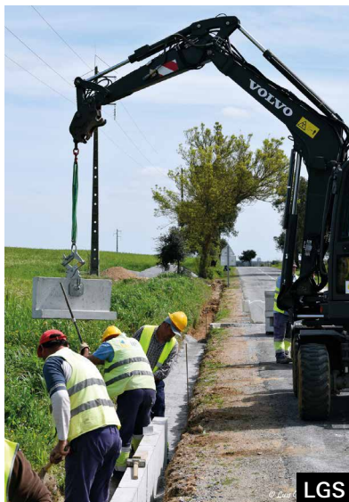
Installation of the permanent concrete barriers on the road verges.
