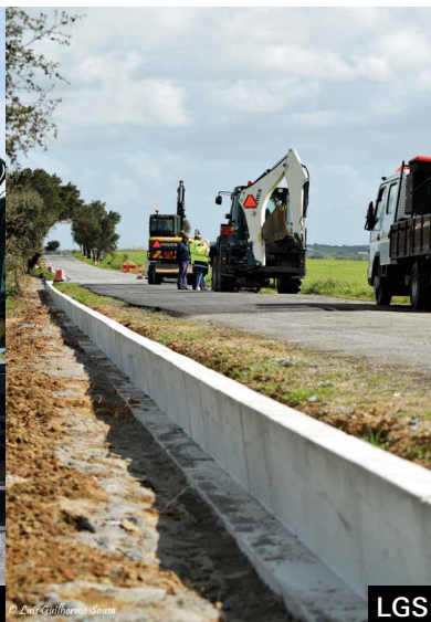
Installation of the permanent concrete barriers on the road verges.
