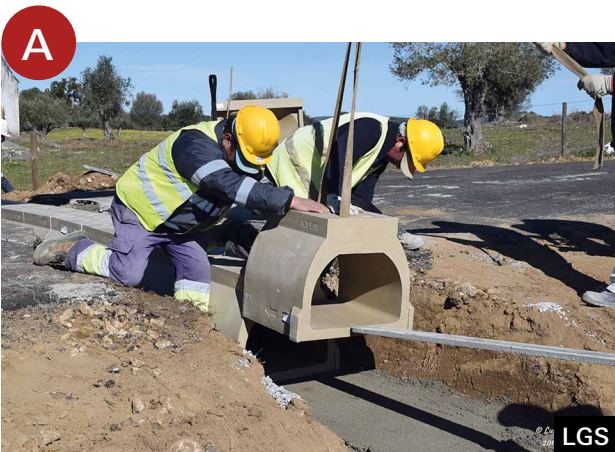
Adaptation and integration of a circular culvert with a permanent concrete barrier.
