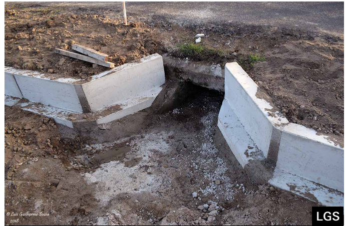
Works to implement permanent concrete barriers guiding animals towards the culvert.
