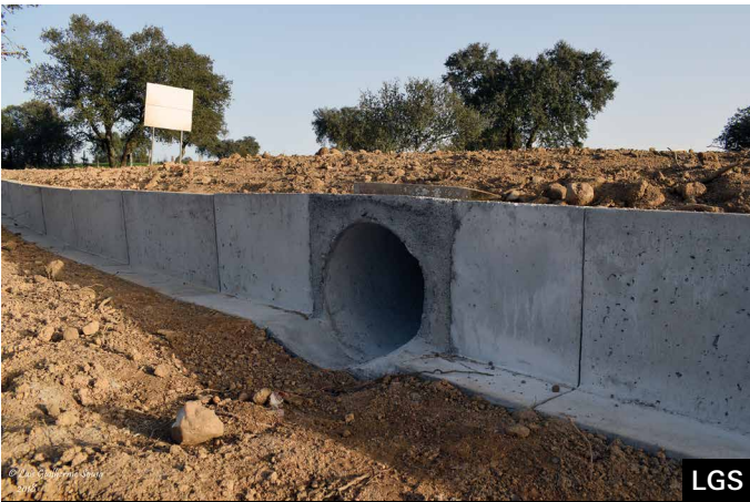
Adaptation and integration of a circular culvert with a permanent concrete barrier.
