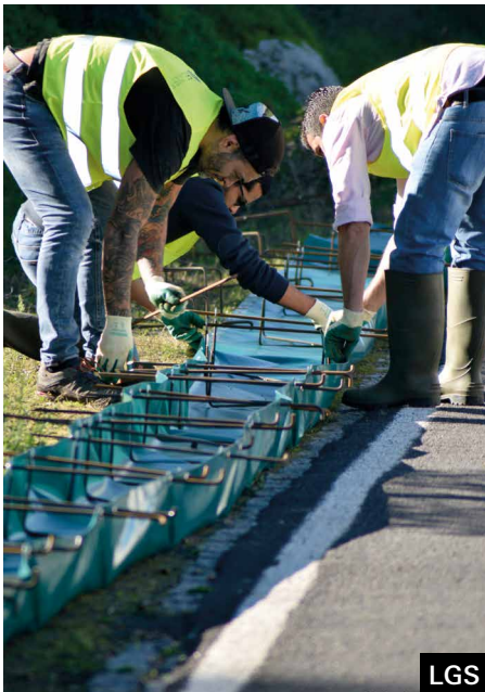
Installation of the temporary canvas barrier in the framework of the LIFE LINES project: (A) placement of the support structure, and (B) final aspect of the installed barrier.
