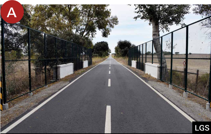
Examples of wire mesh barriers installed during the project: (A) municipal road 529; and (B) national road 114.
