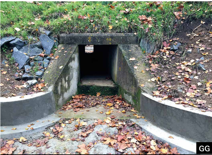
Adaptation of a rectangular culvert in the framework of the LIFE LINES project, by creating an entrance ramp and connecting it to the guiding barriers.
