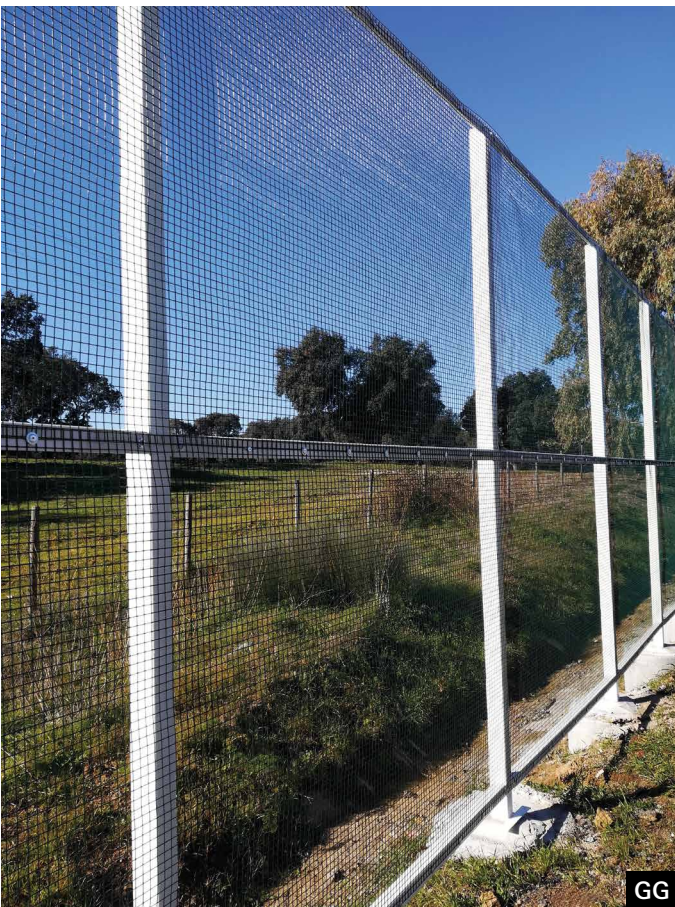
Details of the 3 m-high barriers implemented on the national road 114 road, made of rectangular-section metallic posts (RHS 80x60x3 cm) inserted in the foundation and topped by plastic caps, 2 m apart, that support a galvanised wire mesh welded and plasticized with PVC/polyester, with a 19 x 19 mm of diameter and a wire diameter of 2 mm.
