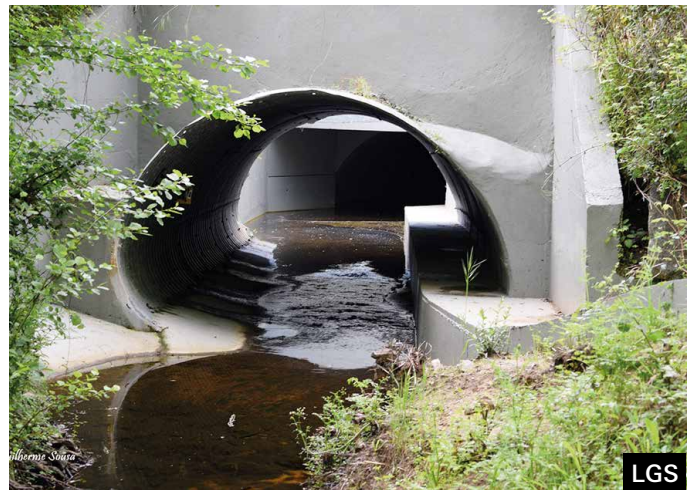
Building of the dry ledge and final aspect, in one of the culverts where this solution was implemented.
