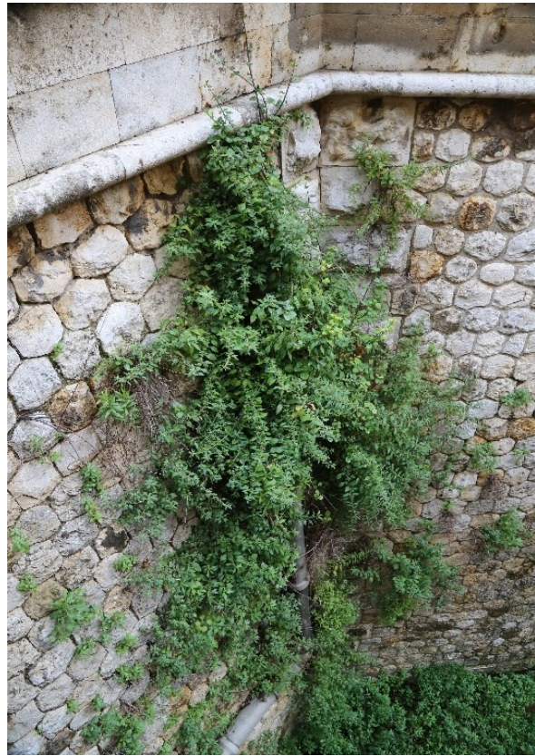
Fig. 4- Nitrophilous casmophytic vegetation ( Parietaria judaicae ) on the wall of Castello fortification realized with exagonal ashlar of limestone
