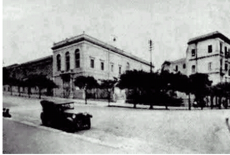
Fig. 1- View of Tobacco factory masonry of “Monopolio di Stato” (Cagliari)
