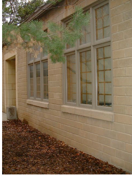
FIG. 2. CSSB construction done in 1943 Broadcast Hall, University of Kansas
