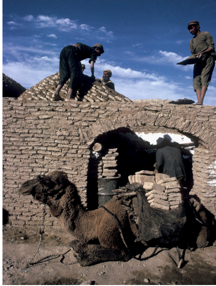
FIG. 1. Traditional mud brick construction Farah Rud, Afghanistan,
