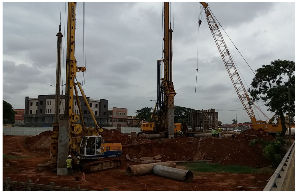
Figure 7. Main view of the Nelito Soares viaduct site and equipment.
