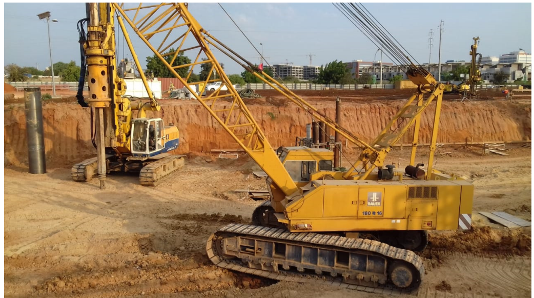
Figure 4. Talatona church site equipment view.
