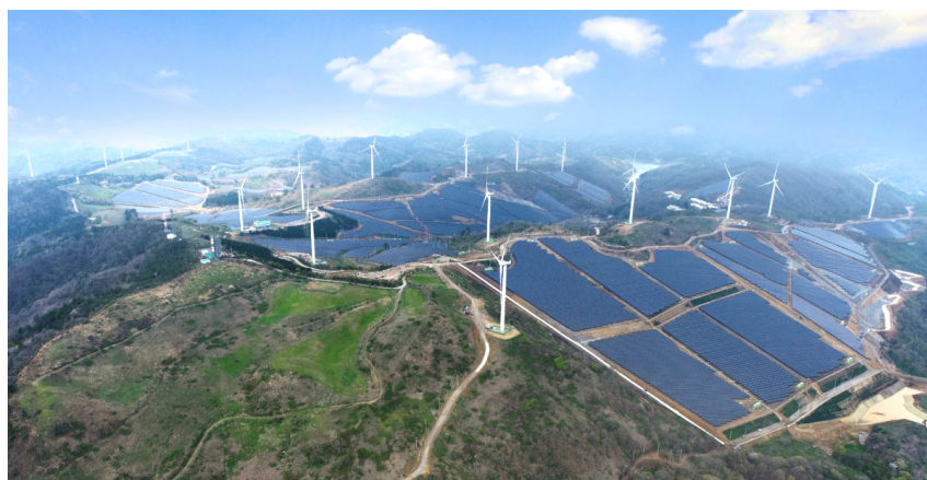
Figure 1.1: Hybrid wind and solar park in South Korea [1]
