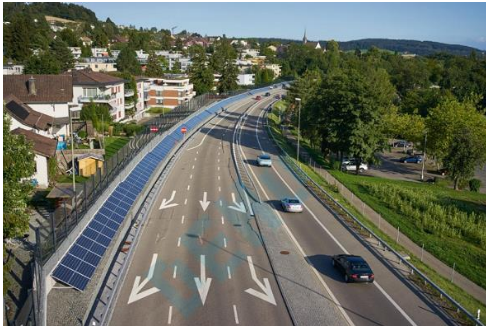
Fig. 23 - PV modules alongside a highway slope [20]
