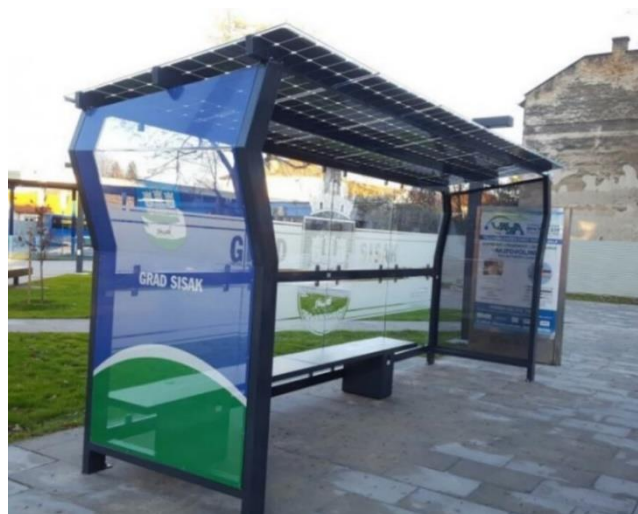
Fig. 284 - Solar PV bus stop shelter in Zagreb, Croatia
