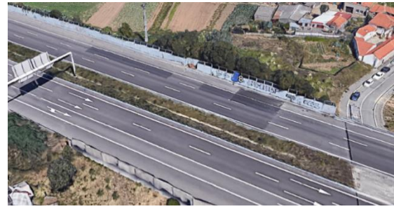
Fig. 44 - Site 8, sound barrier
