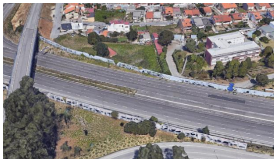
Fig. 45 - Site 9, sound barrier
