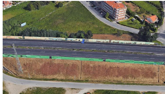
Fig. 54 - Site 18, sound barrier
