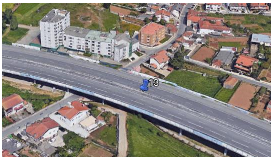
Fig. 49 - Site 13, sound barrier
