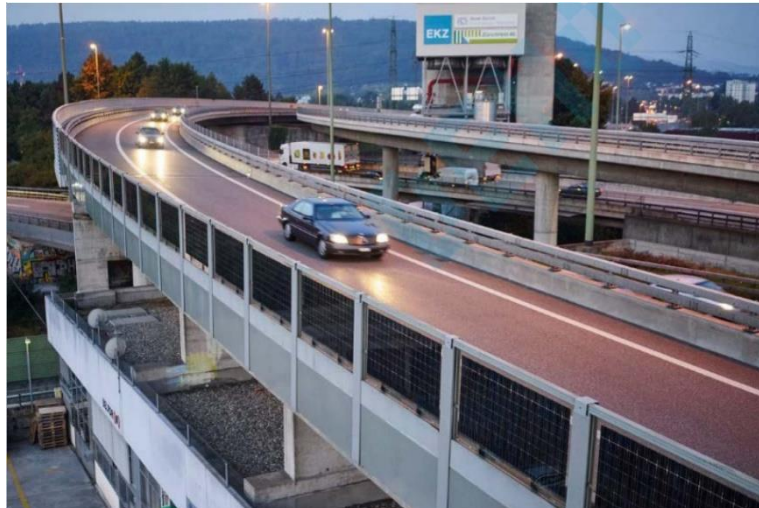
Fig. 25 - Bifacial PVNBs allow light to enter from both sides [20]
