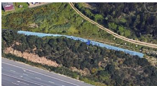
Fig. 37 – Site 1, sound barrier
