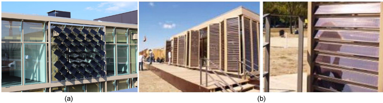
Fig. 3 Different PV shading devices, (a) with a more aesthetical approach (Jayathissa et al. 2017; reprinted with permission ©2017 Elsevier) and (b) with louvers design (Kang et al. 2012; reprinted with permission ©2012 Elsevier)
