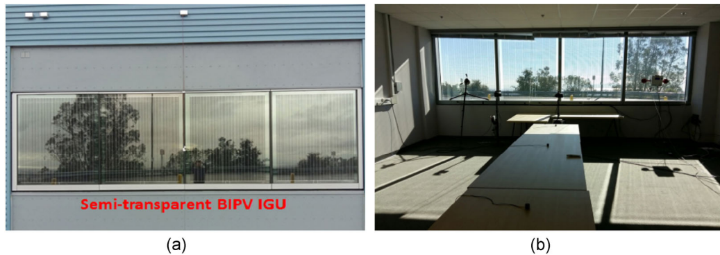
Fig. 2 (a) External view and (b) internal view of the BIPV IGU consisting of narrow c-Si cell strips (Peng et al. 2019; reprinted with permission ©2019 Elsevier)
