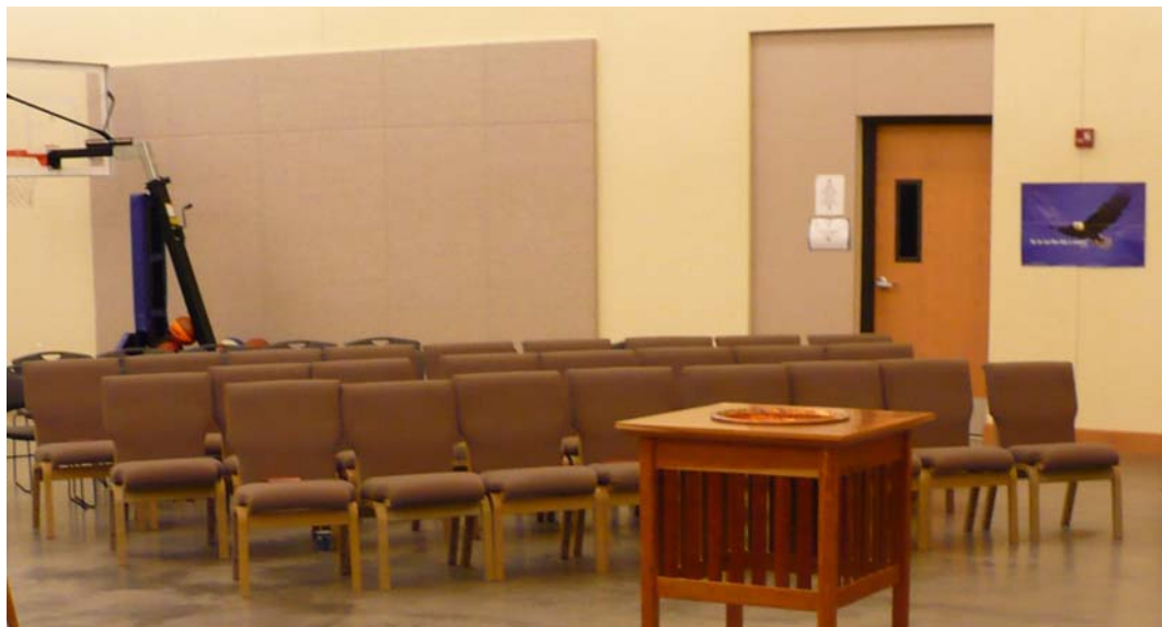
Figure 6-7: Multipurpose Room Absorptive Seating
