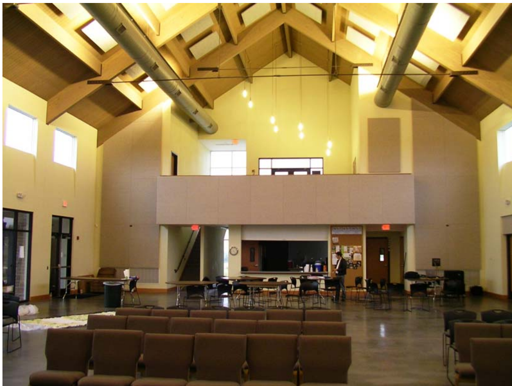
Figure 6-5: Multipurpose Room with Added Absorption on North Wall
