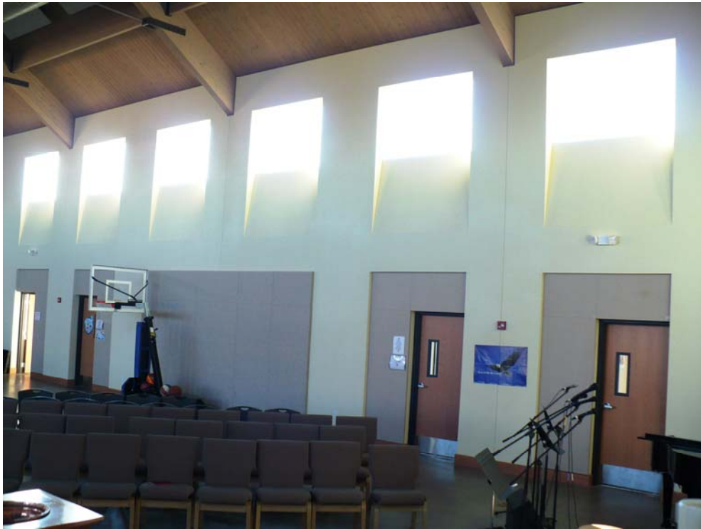
Figure 6-6: Multipurpose Room East Wall with Additional Absorption
