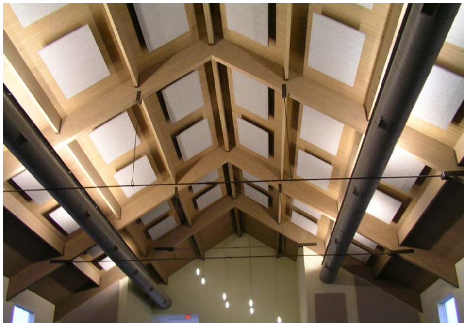
Figure 6-4: Multipurpose Room Suspended Tectum Ceiling Panels
