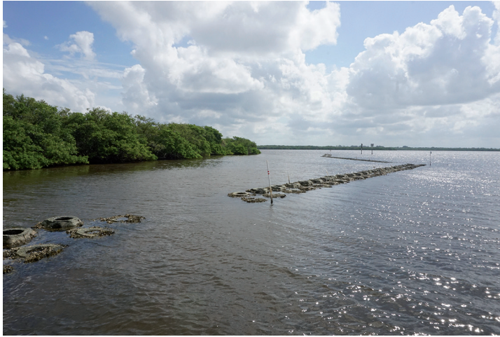
Figure 13. Wave attenuation devices on the north side of the island. Image by Brian Cook.
