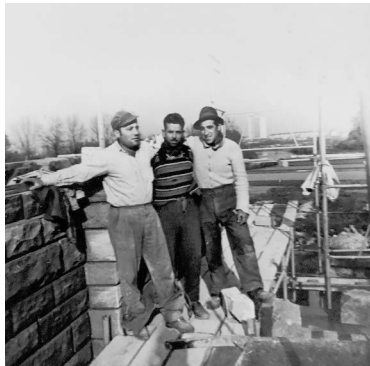
Figure 35: Construction workers posing on top of a scaffold
