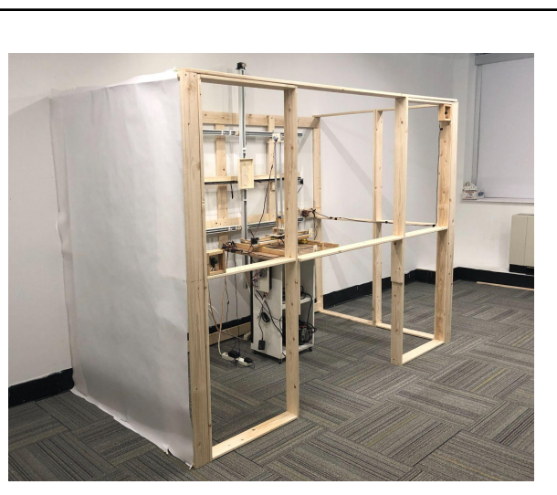
Figure 2. Installation prototype, Structure View 2. 2022
