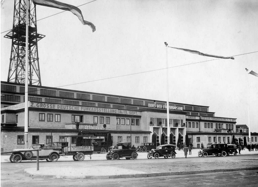
Figure 1.3. Haus der Funkindustrie with the broadcasting antenna in the background (1925). Source: ullstein bild.
