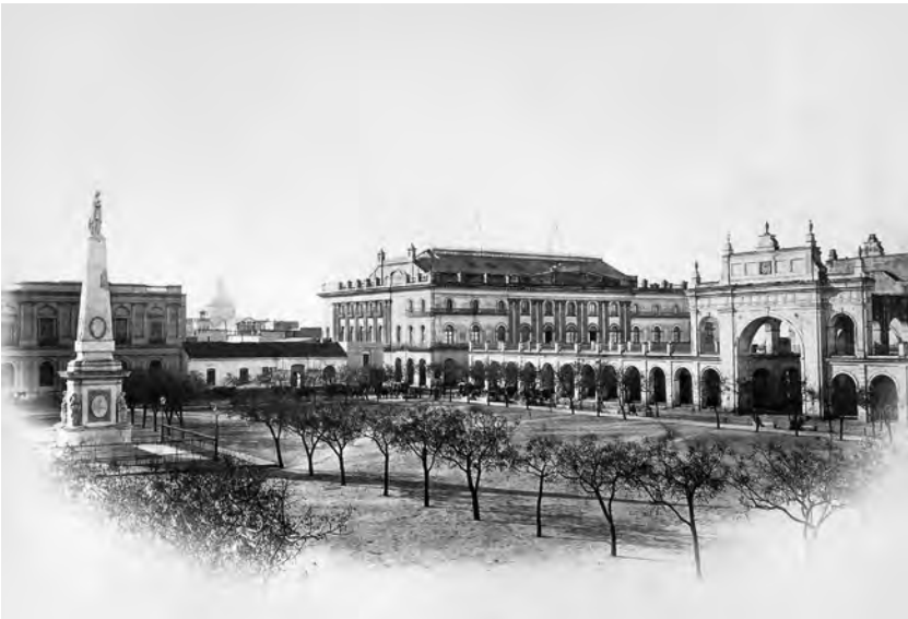
Figure 30. Benito Panunzi, The Pyramid and the Recova Vieja , 1867. Carlos Sánchez Idiart collection, Buenos Aires. The view is taken from the opposite side of the square. Note the transformation of the walk executed by Pueyrredón, with its trees and iron fences, as well as the new profile of the pyramid, now crowned with the statue of the Republic-Liberty and four statues at its base, following Joseph Dubourdieu's design.
