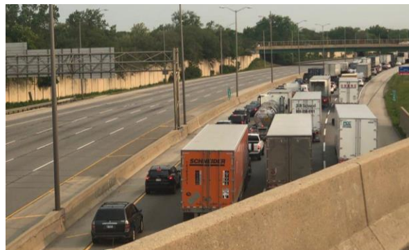
Figure 2-4. Heavy Truck Traffic on I-294, near accident site
