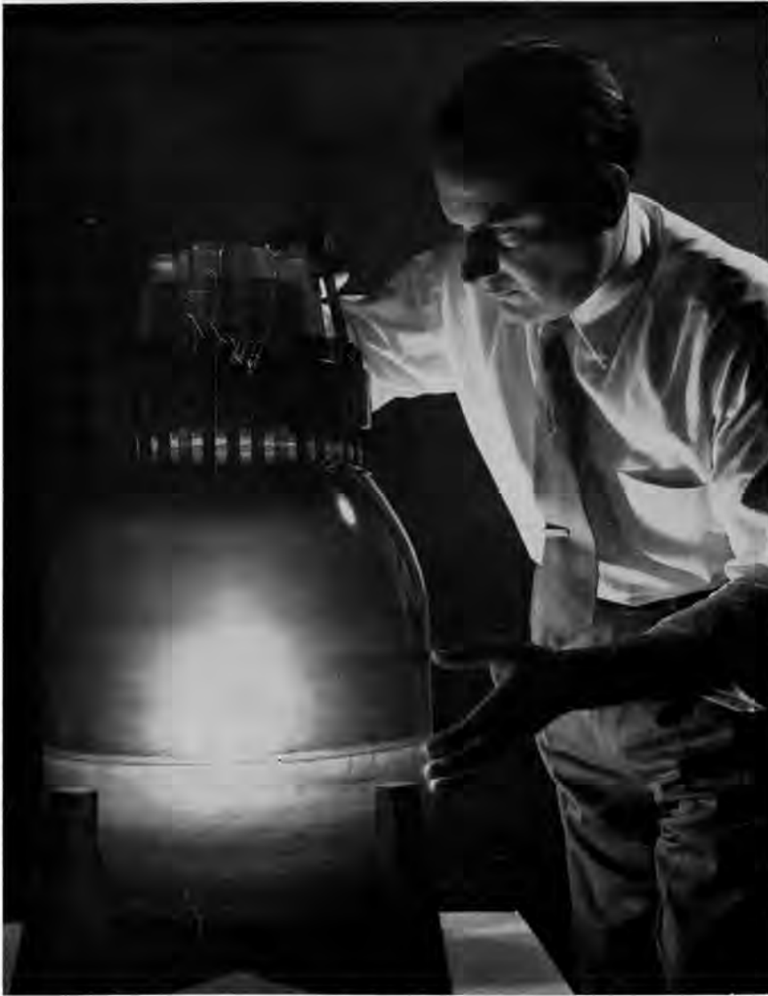
GLOWING 'SHELL' OF NUCLEAR REACTOR —This glowing model enables scientists at the Westinghouse Research Laboratories to study the stresses deep inside the pressure vessel, or "shell," of a full-scale nuclear reactor.
