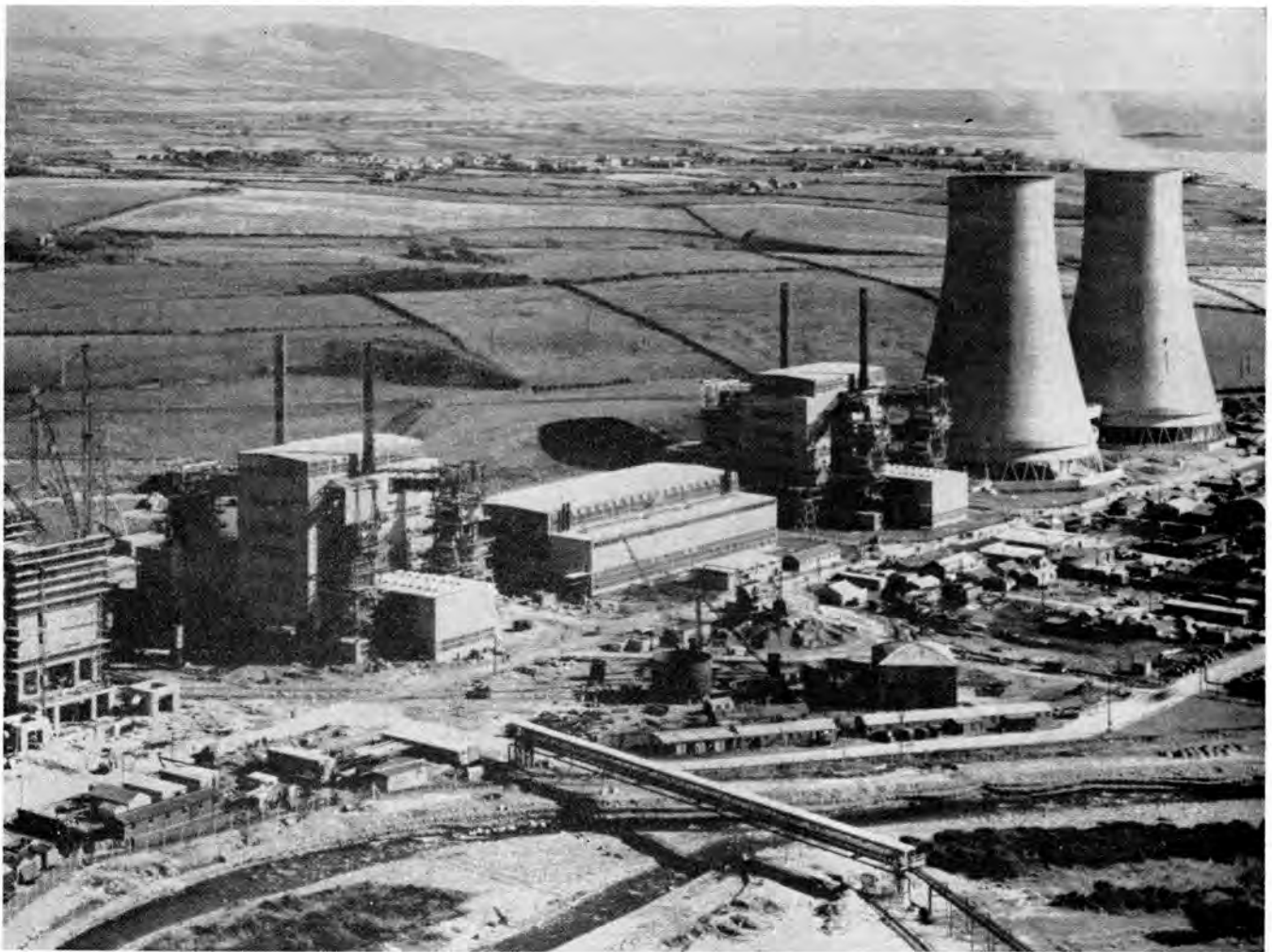
Britain's Calder Hall, the first large scale atomic power station, is already in use. Built in just over three years, the Calder Hall station uses atomic energy to produce electricity for homes and factories in Britain. Shown in the center are the power house and reactors (heat exchanger outside). At the far right are the cooling towers.
