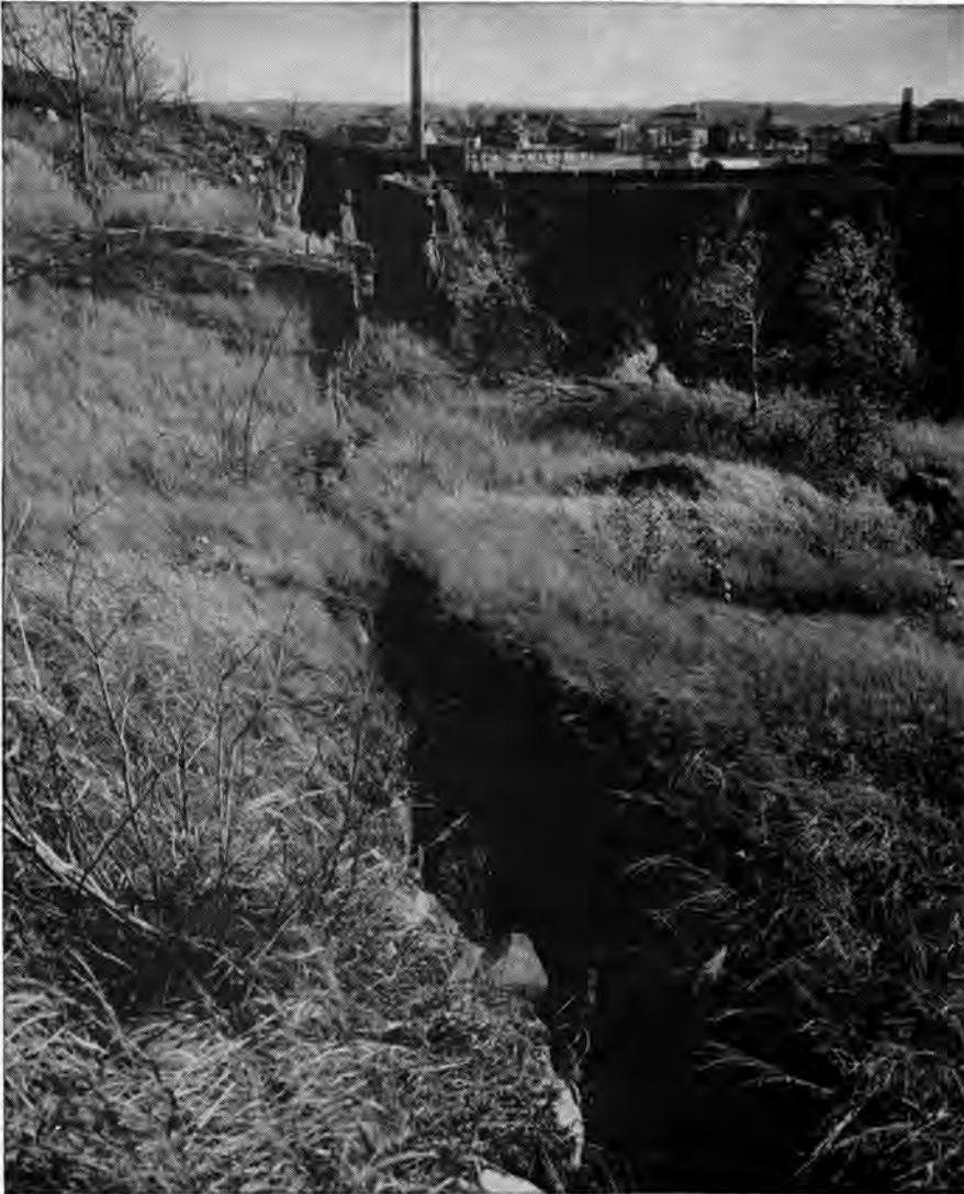
A crack at the earth's surface shows bulk mining is proceeding far underground.
