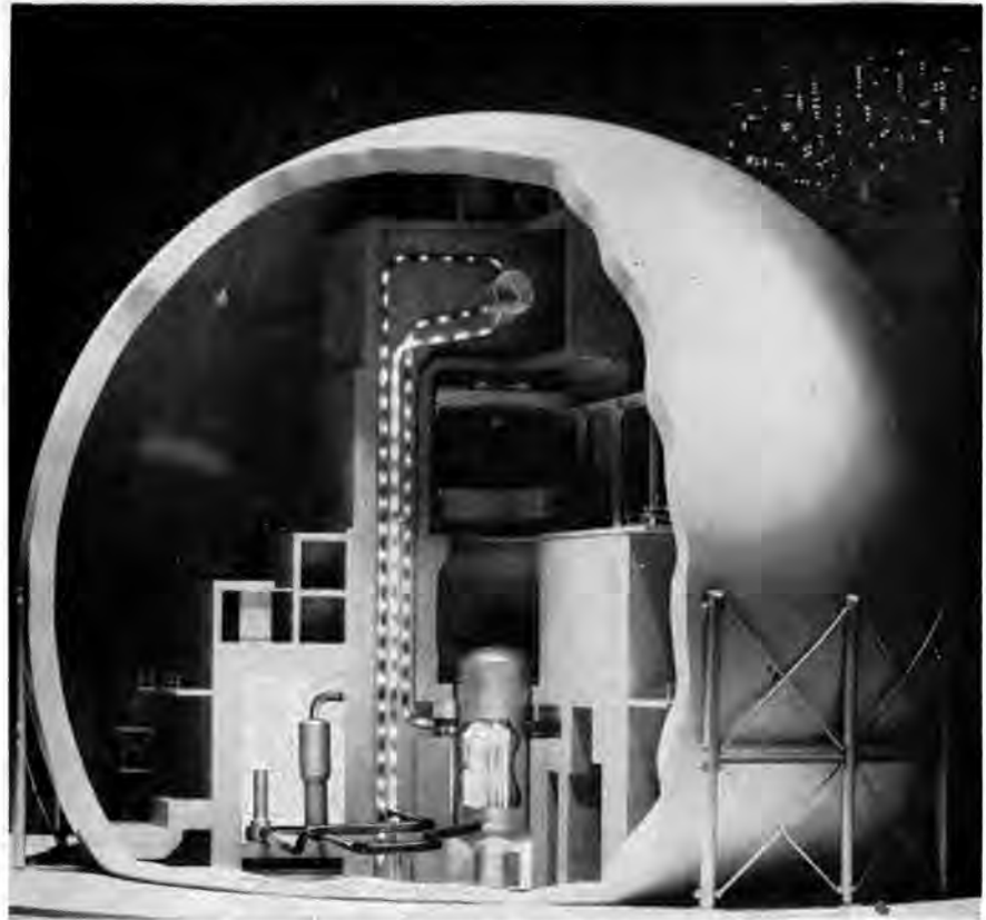
A model of the dual cycle boiling water reactor. The reactor package is shown in section view revealing interior details. The steel sphere housing the reactor is 190 feet in diameter.
