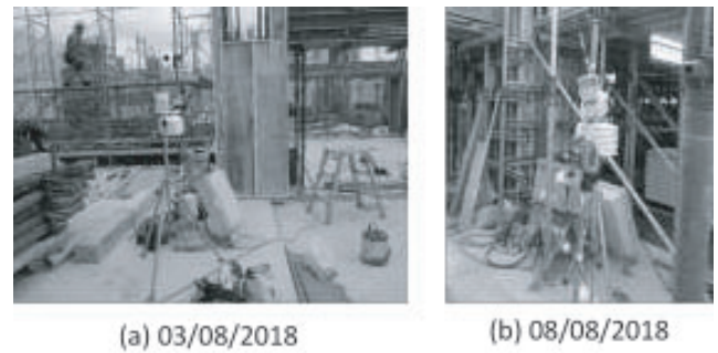
A On the sixth floor for form workers
