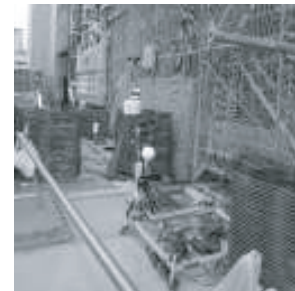
B On the ground for rebar placer
