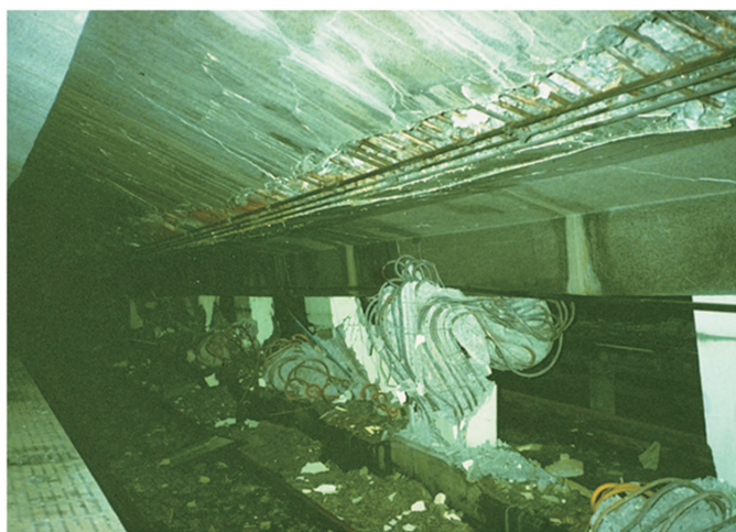
Fig. 2. (Color) Compression failure of the central columns of the Daikai Station subway structure. (Reprinted with permission from Sakurai 2014.)
