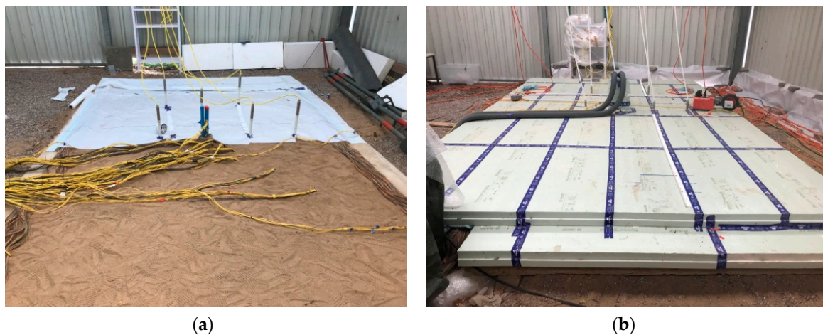
Figure 1. A meso-scale 5 \times 3 \times 2 \text{ m}^3 experimental indoor high-temperature borehole thermal energy storage (BTES) of project Angus II in Kiel, Germany, with a cemented closed loop borehole heat exchanger (BHE), containing dual u-tube pipes, located at the center of the heat storage system: (a) installation of sensors in the heat storage soil, a fine-sand, which is one of the subjects of investigation of this research; (b) the heat storage system after insulation.
