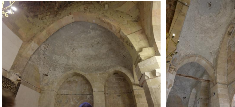
Figure 5: Brick vaults adjacent to the western façade of the mosque section
