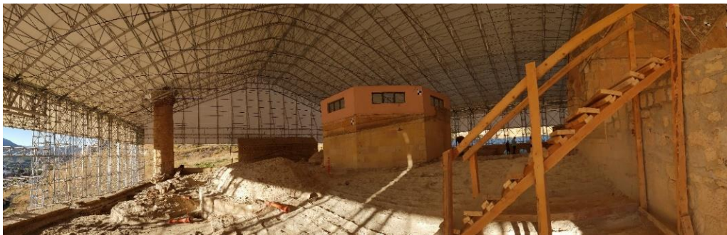
Figure 18: Temporary roof structure for protecting the structure during the restoration works
