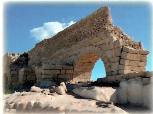
Water was provided for Caesarea Maritima by an extensive system based on this Herodian aqueduct.
