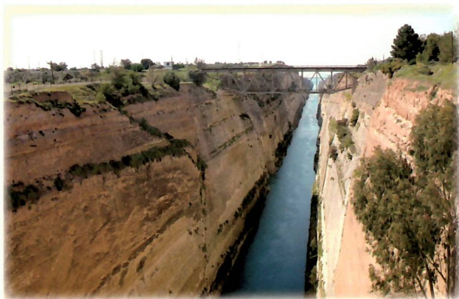
Corinthian canal. Nero brought 6,000 Galilean slaves to work on the canal, but the project stopped at his death. The canal—four miles long and seventy-five feet wide—was completed between 1882 and 1893 and connects the Gulf of Corinth with the Aegean.
