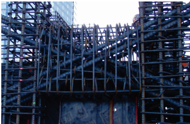
Figure 1 - Diagonally reinforced coupling beam
