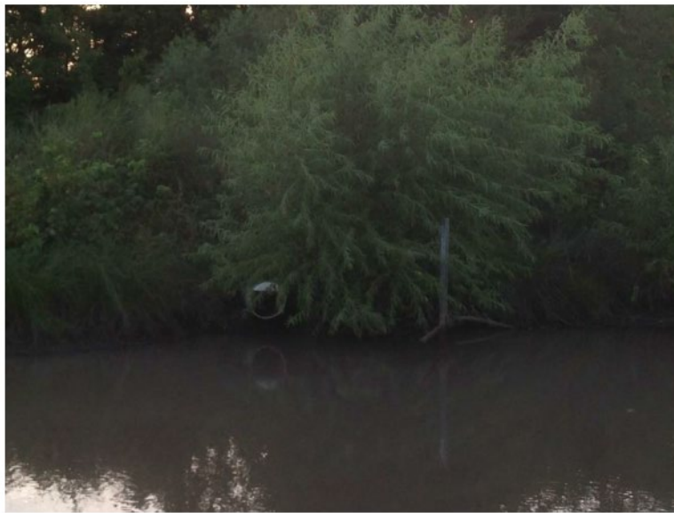
Fig 1. 6 Outflow pipe for Cain wetland, Picture taken in July, 2017, from [33]
