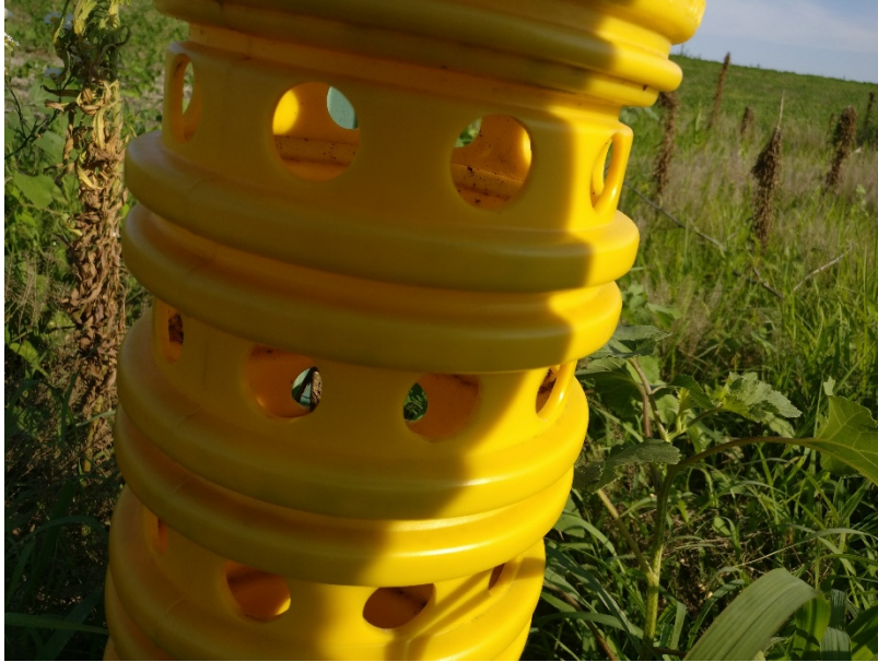
Fig 2. 5 Standpipe riser photograph
