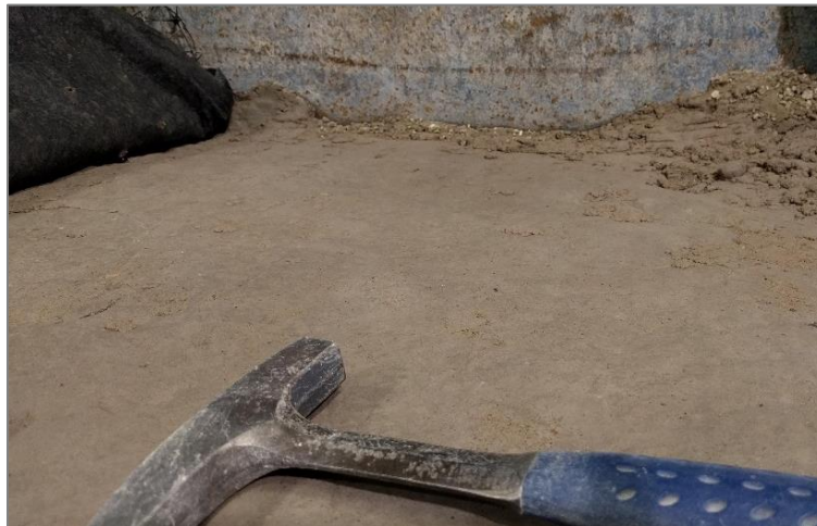
Figure 4.3. Subgrade Surface in the VGB/GG/NW Section after Loading and Excavation.
