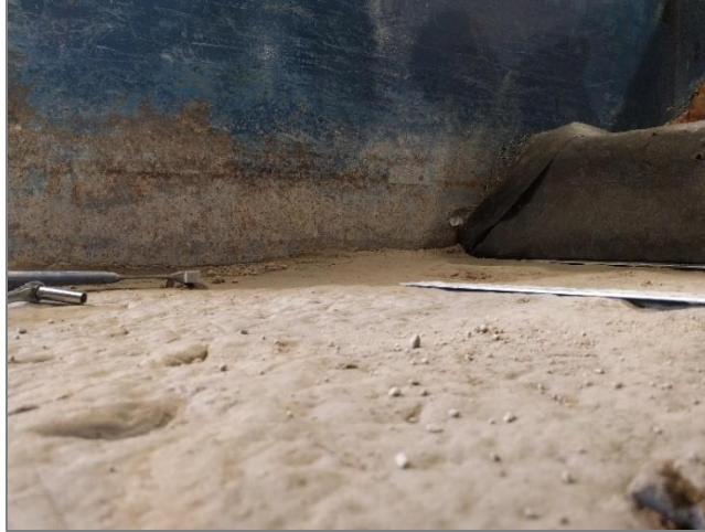
Figure 4.4. Subgrade Surface of the RCA/GG/NW Section after Loading and Excavation.
