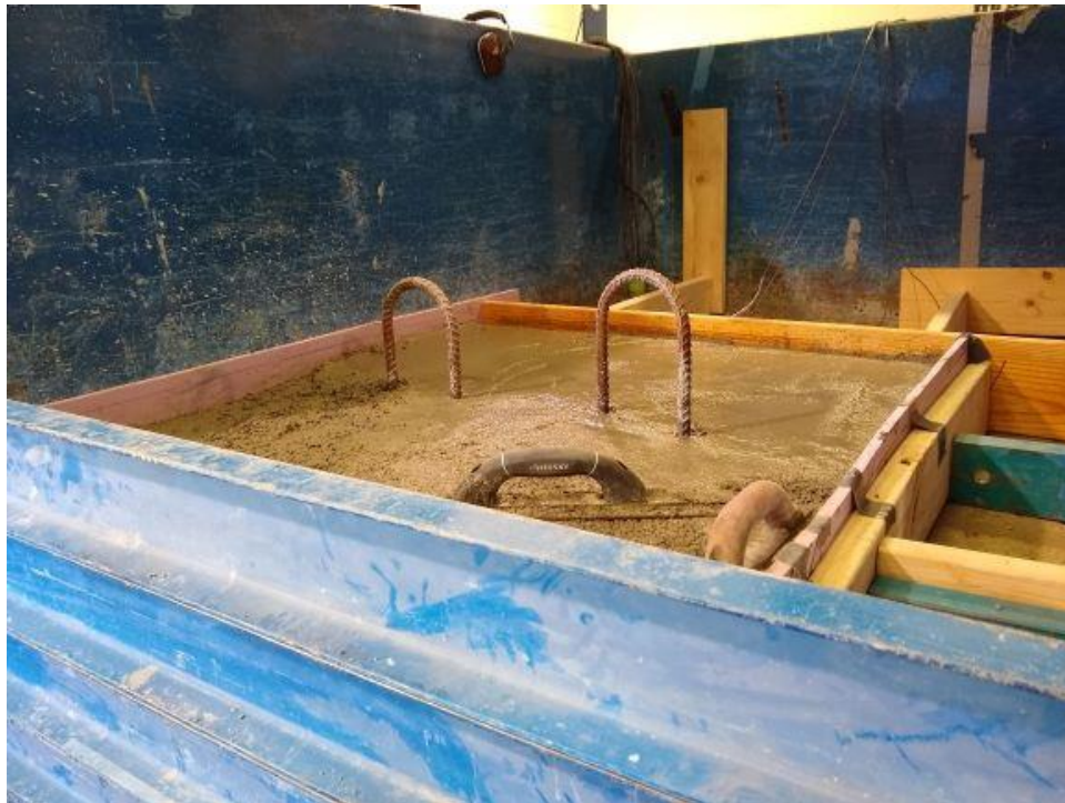
Figure 3.23. Loaded Concrete Slab During Pour and Compaction.
