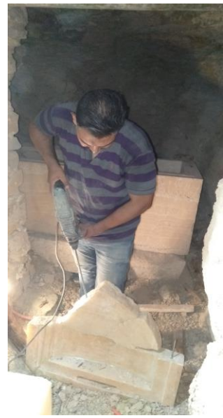
Fig. 9 During the drilling in third part
