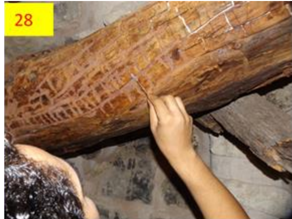
Photo 27-28 Filling on the cotton by using microballoon with a suitable color mixed with B72 15% after ensuring that the color of the filling matches the wood
