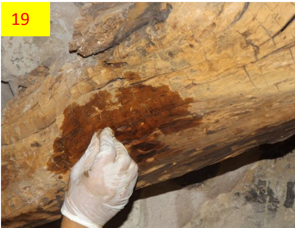
Photo 17-20 Mechanical and chemical cleaning
