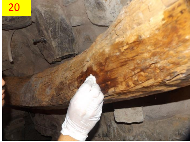
Photo 17-20 Mechanical and chemical cleaning
