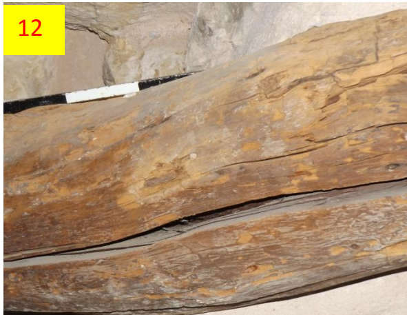
Photo 10-13 Deterioration forms on wood trunks
