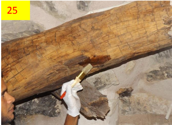
Photo 23-26 Injection by using B72 20 to harden the cotton, consolidating wood by using Plexisol P550 3-5-7% and making a test of filling on the cotton by using microballoon with a suitable color mixed with B72 15%
