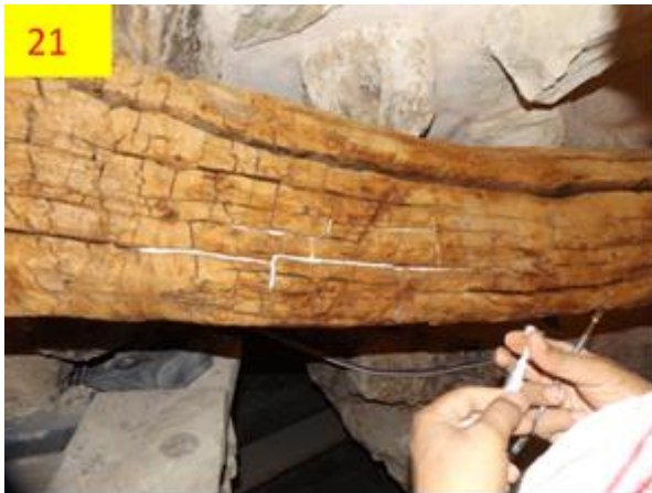
Photo 21-22 Filling among cracks by using cotton
