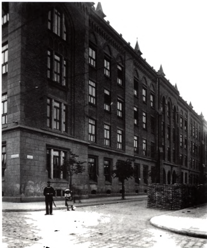
187. Municipal schools at 3/5/7 Wąska Street, by Jan Zawiejcki (1911–1912)
