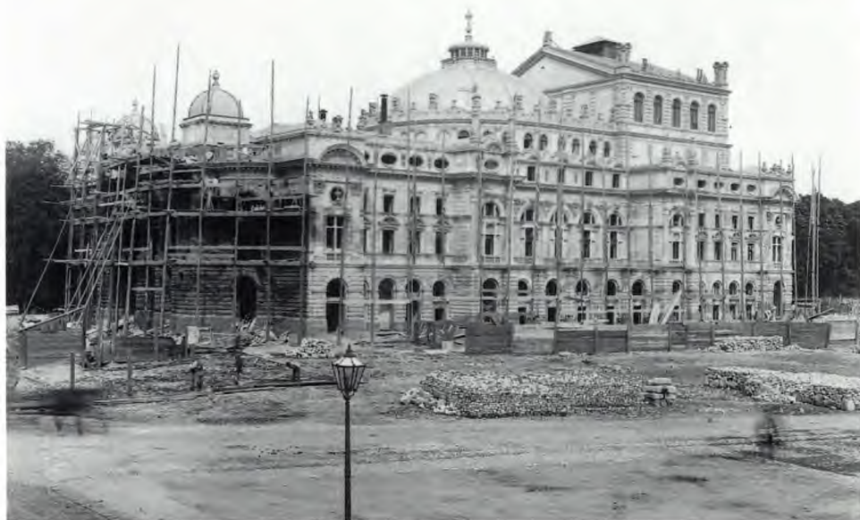
13. Cracow. Municipal Theatre during the finishing work, 1893
