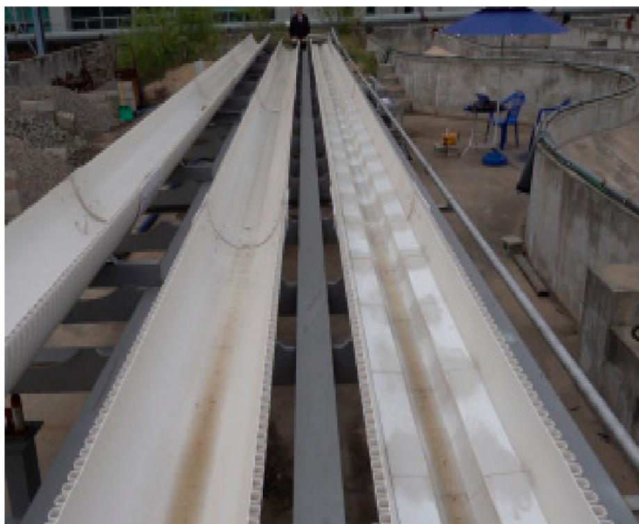
Figure 8. Transportation of the sediment on the experimental sewer pipe lines.
