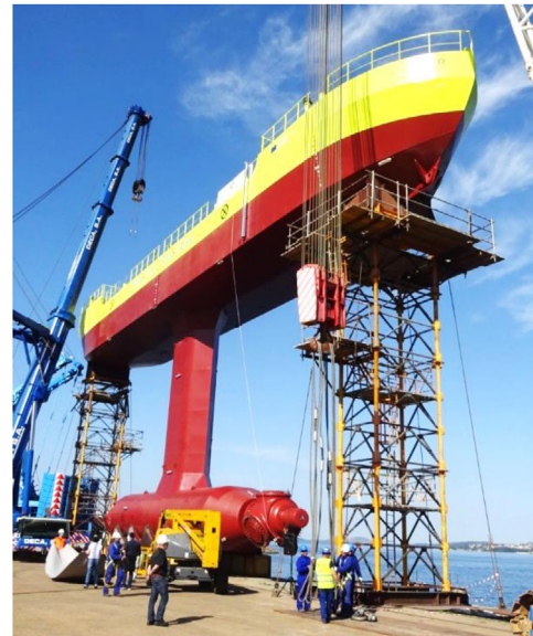
FIGURE 2 Platform launching in the harbour of Vigo
