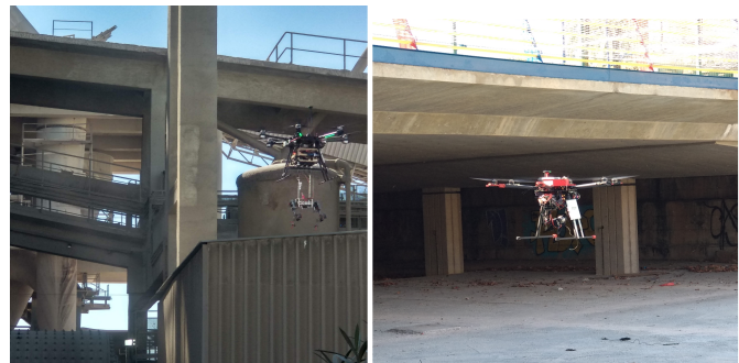
Fig. 1. Pictures of SNSR validation experiments in status monitoring of a bridge (right) and a cement kiln (left), location omitted for confidentiality.
