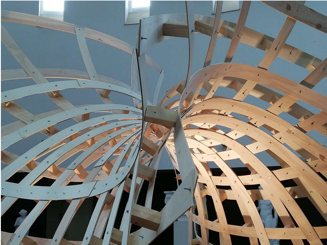
Fig. 11 Detail of the double-layered shell of the pavilion. The continuity of the strips is solved by overlapping, taking into account the continuity of the geometric curvature of them. Images: authors
