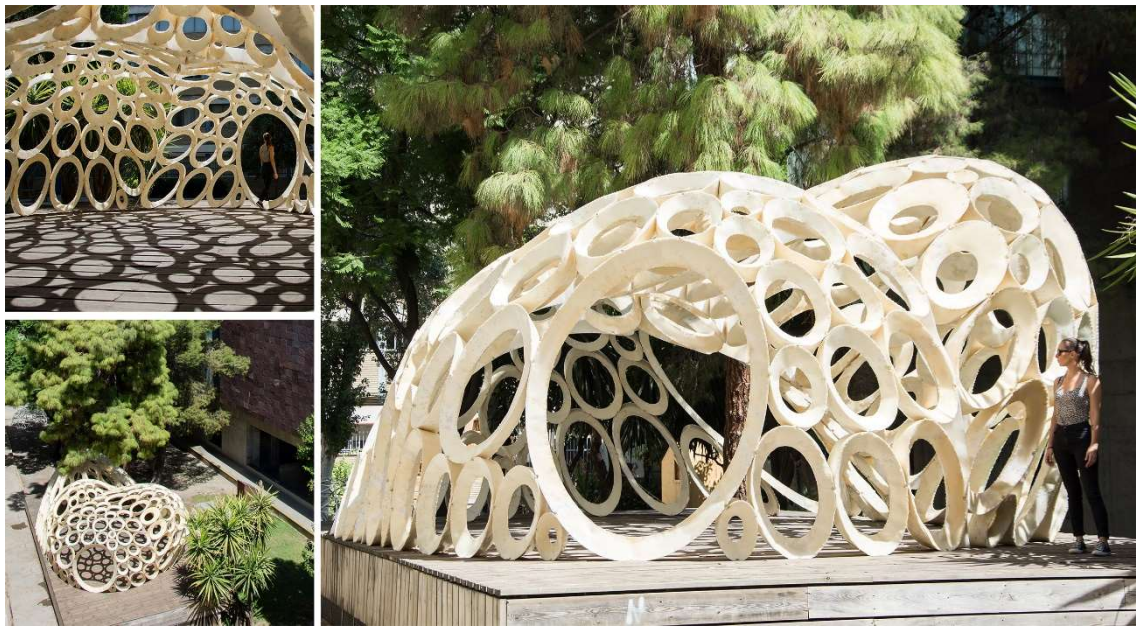
Fig. 19. Photographs of the Archimedean Pavilion (by Roberto Narvaez-Rodriguez), 2016, composed of four inclined rotational paraboloids which were discretised with an algorithm based on the initial property stated by Archimedes. Source: Authors' own
