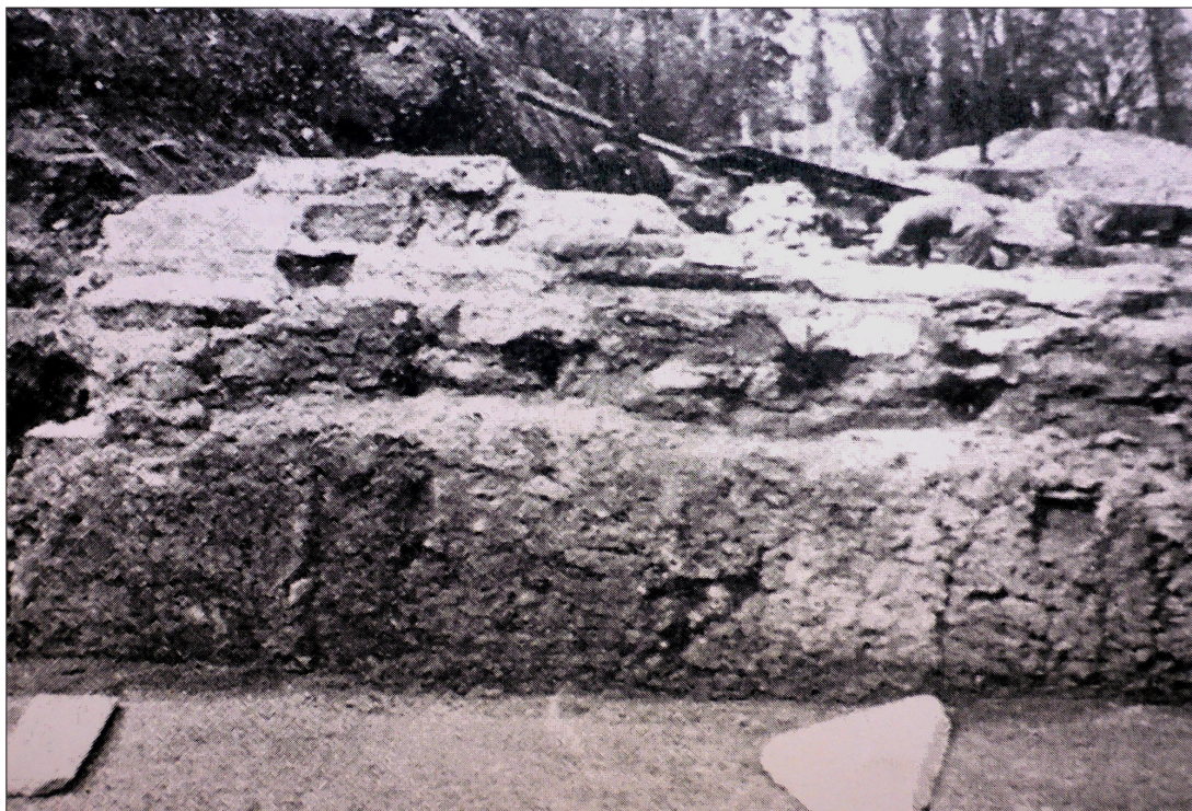
Fig. 11. Imprints of marble plates in mortar and the place of iron clamps in the wall (PAULOVICS 1943, 13. kép).
