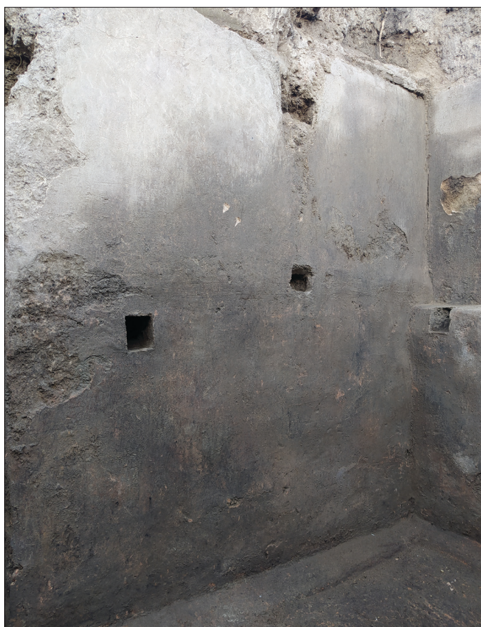
Fig. 9. Beam cavities in the cellar.
