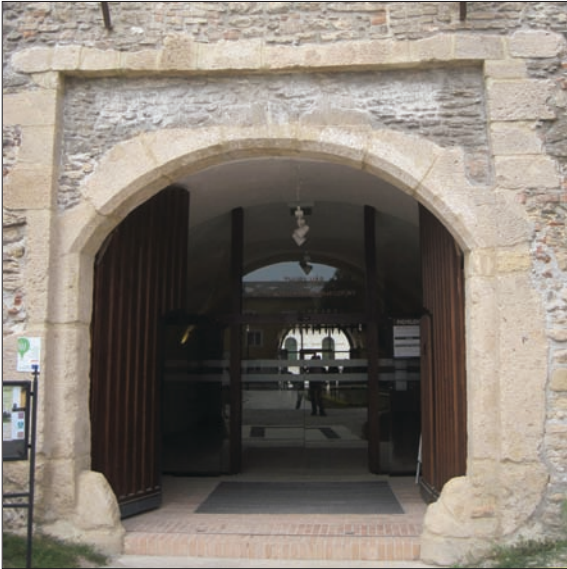
Fig. 7. Gate of the southern gate house with traces of the draw bridge (Várpalota Castle).
